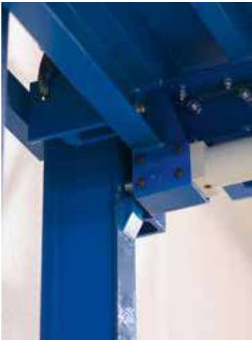
Details of the anti-creep latch
